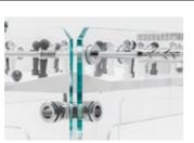
NO GLUE NO ELEMENT IS GLUED TO THE GLASS, BUT EACH PIECE WAS ATTACHED THROUGH JOINTS MILLED FROM SOLID.
